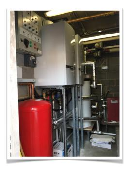
A condensing boiler captures much of the heat in the exhaust gas from a boiler and improves the efficiency by ~11%. Gas boilers can thus race over 90% efficiency.
